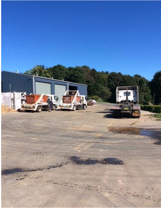
Figure 5: Existing Shed 2 (facing west)
