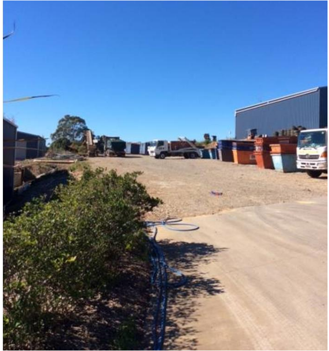
Figure 6: Site of proposed Shed 4 (facing east)
