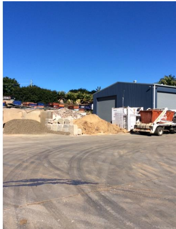
Figure 10: Existing Shed 2 (facing west)
